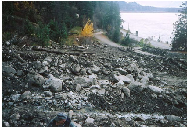
D) Debris on Kuskonook fan-delta. Maximum boulder size reported to be 1 m. D. VanDine photo.
