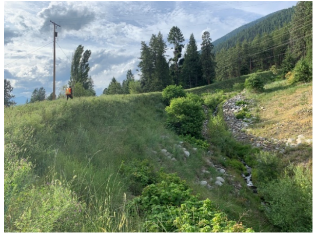
B) Standing on berm looking upstream (north) showing rip rap at the base of the berm.
