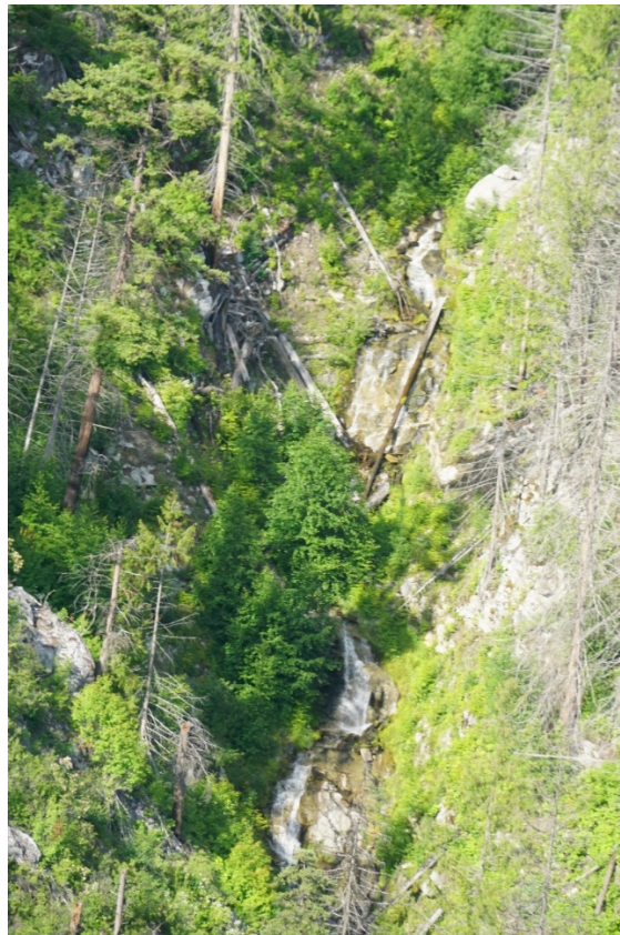
Figure 6-1. Channel of Kuskonook Creek in mid reaches (elevation ~ 1300 m) with bedrock sections alternating with coarse angular debris. Photo: BGC, July 7, 2019.
