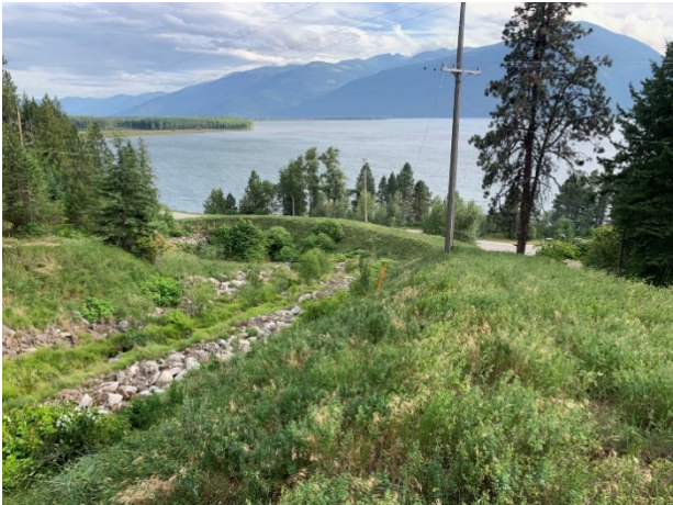
A) Standing on berm looking downstream (south) showing rip rap at the base of the berm.
