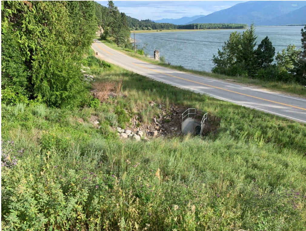
Figure 3-5. Spillway culvert crossing Highway 3A at Kuskonook. BGC photo taken July 10, 2019.
