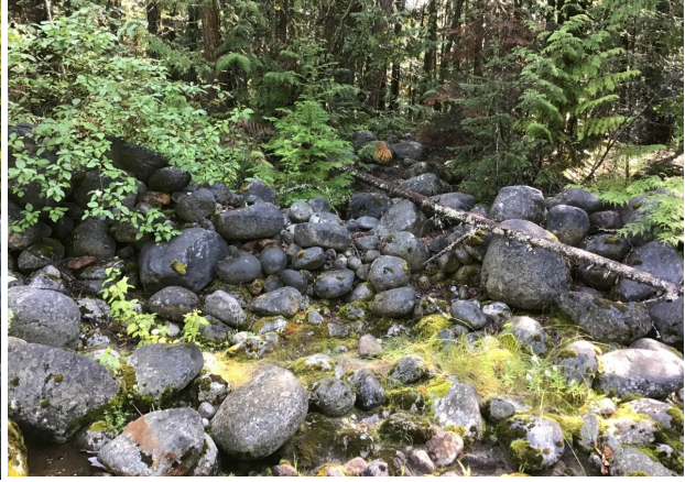
B) On the left bank looking east at the low point along KKN-FP-02, approximately 90 m upstream of the Highway Bridge.
