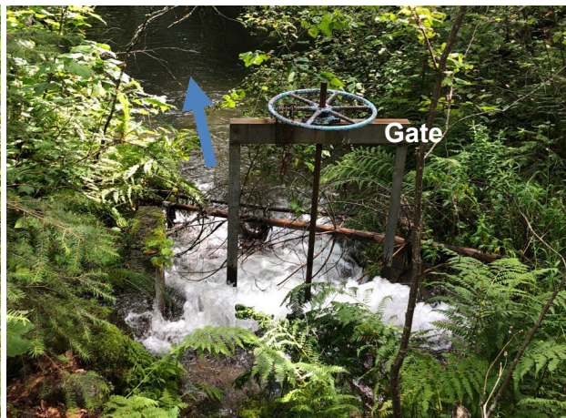
B) On trail, looking south and downstream at gate controlling flow into the Fish Spawning Channel.
