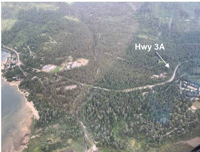
Photo 2. Overview photo taken during helicopter overflight looking north at the Kokanee Creek fan with Hwy 3A (left to right) running across Kokanee Creek. Photo: BGC, July 6, 2019.
