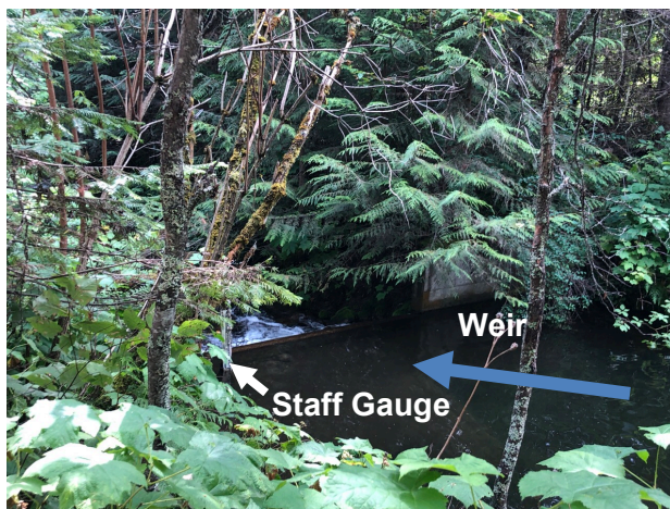
C) On the left bank looking south-west and downstream at weir and staff gauge for measuring flow in Fish Spawning Channel.
