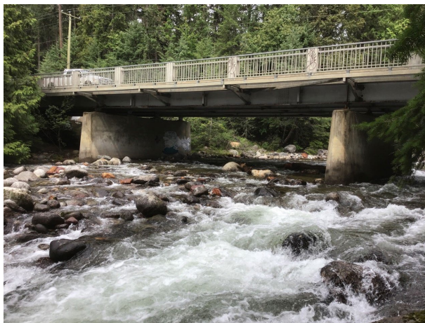
B) On downstream left bank looking upstream at the downstream face of Kokanee Highway Bridge.
