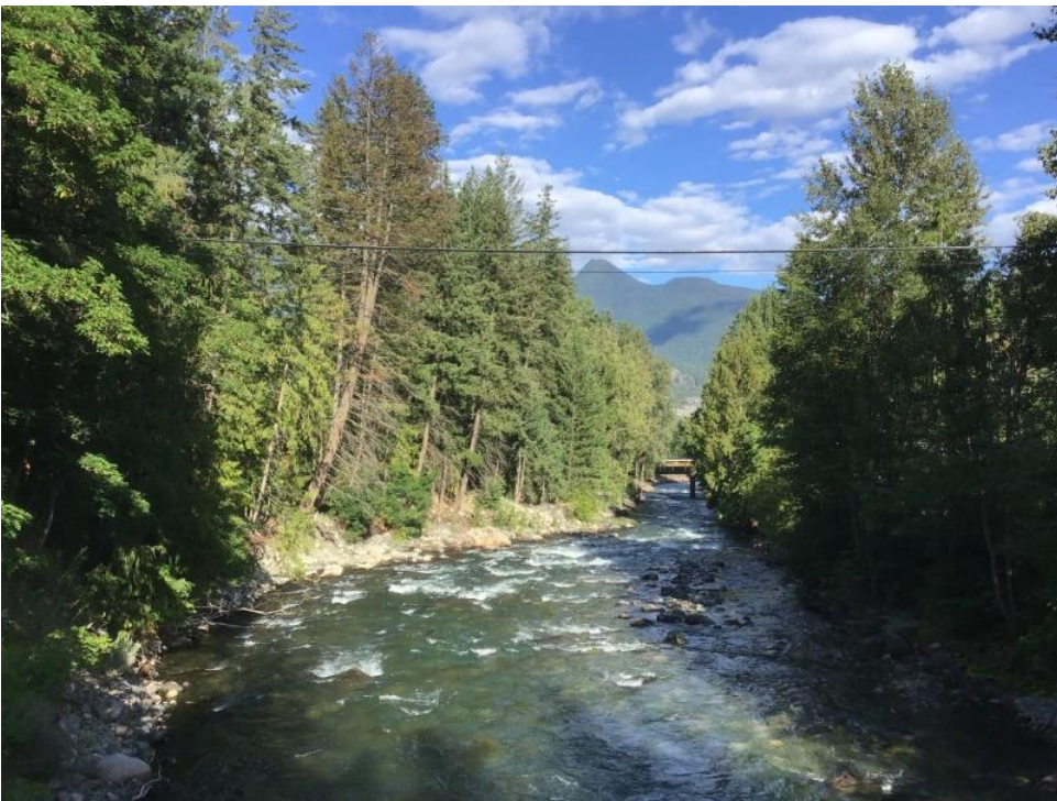
Photo 4. Standing on the Kaslo River Trail pedestrian bridge looking downstream. The Highway 31 bridge is visible in the distance. Photo: BGC, July 4, 2019
