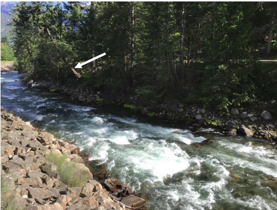
Photo 8. Example of bank erosion. In this location the right (far) bank is eroding causing the leaning tree (arrow) to be undermined. Photo: BGC, July 4, 2019
