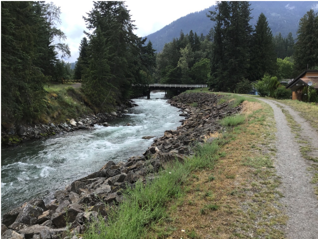
Figure 3-5. Kaslo dike looking upstream towards the Highway 31 bridge. Photo: BGC, July 4, 2019.
