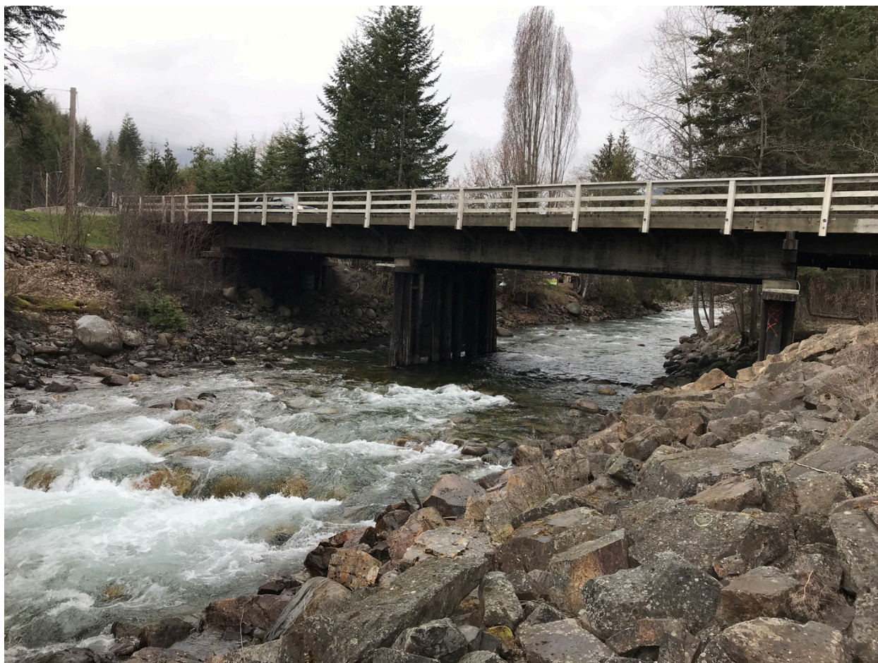
Figure 3-3. Highway 31 bridge over Kaslo River looking upstream (west). Photo: BGC, April 18, 2019.
