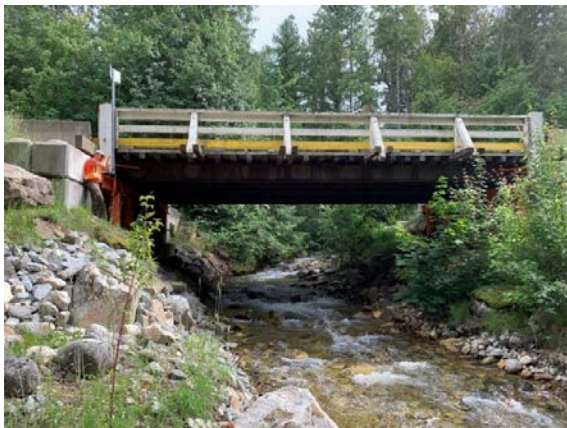
C) Looking upstream (south) at Harrop-Proctor Bridge.
