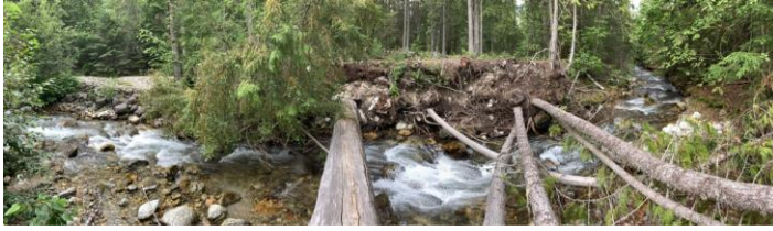
Photo 10. Left bank erosion on outside channel bend of Harrop Creek, approximately 1.35 km upstream of the outlet to Kootenay Lake. Note trees fell across the creek. Estimated age of bank failure 2 years. Photo: BGC, July 2019.
