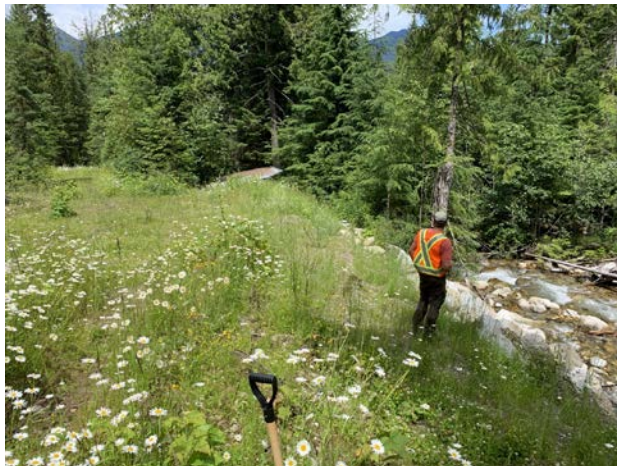
HRP-FP-01 – Rip rap protection on left bank above water intake house (tin roof is visible at end of berm).
