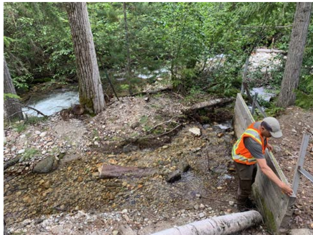
HRP-FP-03 – Water intake with wooden deflection wall (4.10 m x 1.02 m x 0.07 m thick) across avulsion channel.
