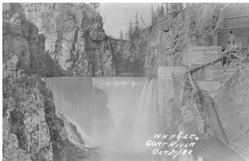
Figure 3-3. Water overflowing the top of the concrete arc dam of the Goat River Dam near Erickson BC in October 1933 (source: Fortis BC Archives).
