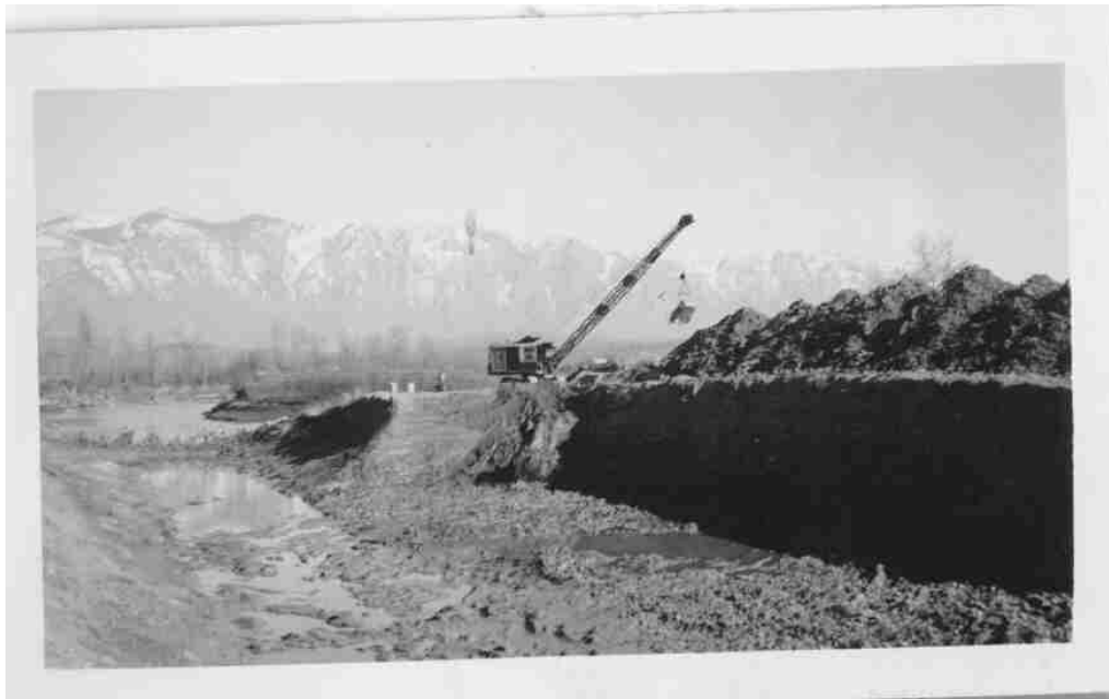
Figure 3-1. 1935 dredging activities at mouth of Goat River.
