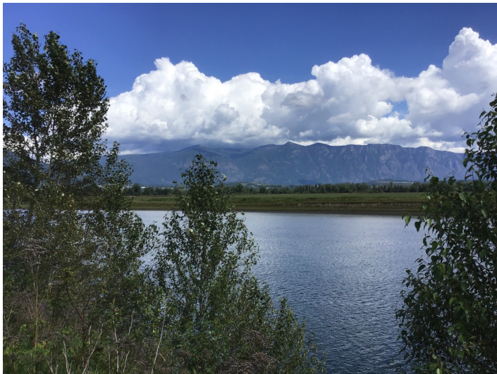
Photo 10. Standing on crest of Kootenay River Dike, approximately 1.5 km downstream of the Goat River's confluence with the Kootenay River, looking across the Kootenay river at the left (southeast) bank. Photo: BGC, July 16, 2019.
