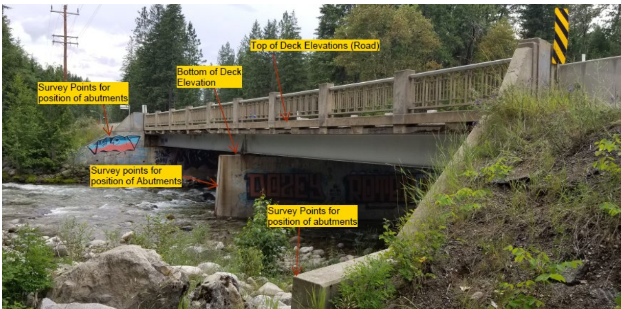
Figure 4-2. Example of bridge structure features collected during the Goat River survey.
