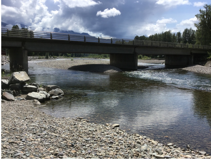
Photo 3. Standing on right bank of Goat River looking upstream (west) at the north Highway 21 Bridge crossing the main channel. Photo: BGC, July 16, 2019.
