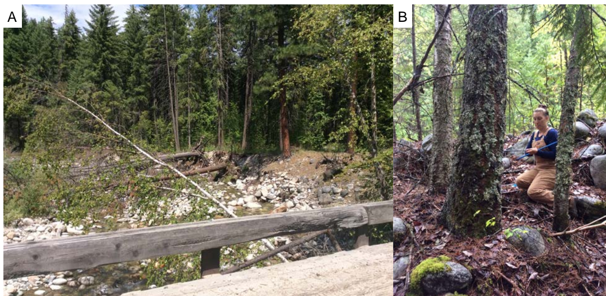
Figure 3-7. Photos of Eagle Creek Dike (EGL-FP-01) near fan-delta apex. A) Looking upstream (north) from Worthington Creek Forest Service Road Bridge at EGL-FP-01 (Photo by BGC July 23, 2019). B) looking south at material of EGL-FP-01 approximately 120 m upstream of the bridge, note the rounded clasts of the dike behind field staff (Photo by BGC July 23, 2019).
