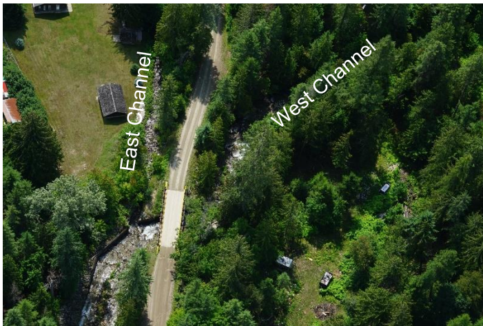
Photo 5. Overview photo taken during helicopter overflight looking down at Duhamel Creek Road Bridge spanning the West Channel and the bifurcation structure. Photo: BGC, July 6, 2019.
