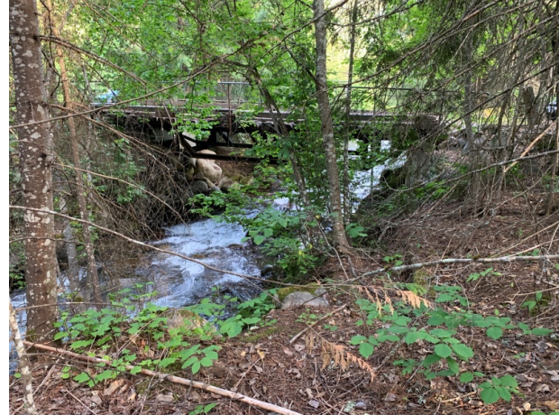
B) Looking downstream at Driveway Bridge 1.
