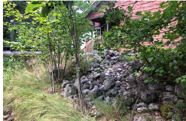
C) DHL-FP-16: Looking at right bank, just upstream of Pedestrian Bridge 2 (left side of photo).
