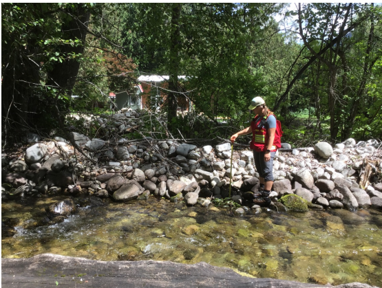
C) DHL-FP-08: Looking at left bank (east), approximately 70 m downstream of Lower 6 Mile Road. Additional berm material visible in the background.
