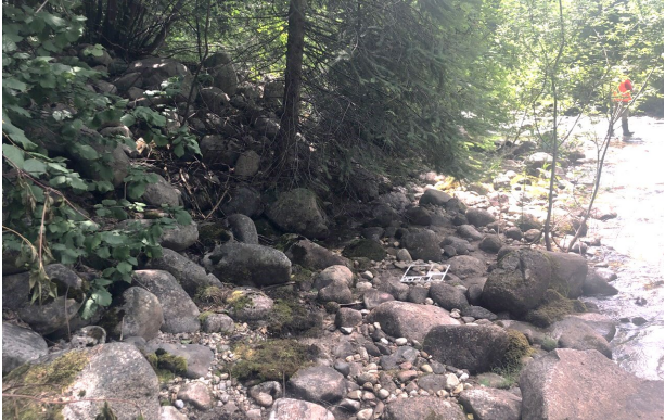
A) DHL-FP-06: Berm constructed of sub-rounded cobbles and boulders approximately 1.5 m to 2 m high on left bank, approximately 50 m downstream of Highway 3A.
