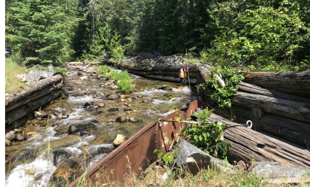
B) Looking upstream (north) at bifurcation with DHL-FP-01 (right), DHL-FP-02 (left), and DHL-FP-03 (center, "V") with Duhamel Creek Rd seen on upper left.
