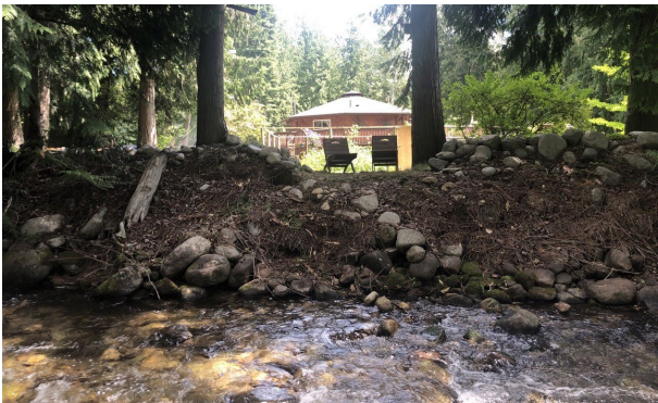
C) DHL-FP-06: Berm constructed of sub-rounded cobbles and old concrete foundation approximately 1.5 m high on left bank approximately 80 m upstream of Lower 6 Mile Road on the western channel.
