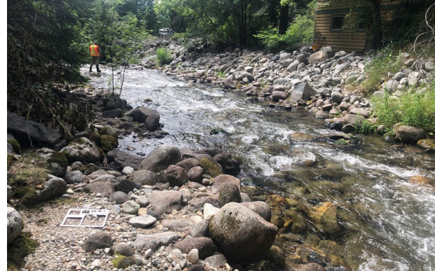
B) DHL-FP-07: Berm constructed of sub-rounded cobbles on the right bank approximately 50 m downstream of Highway 3A.
