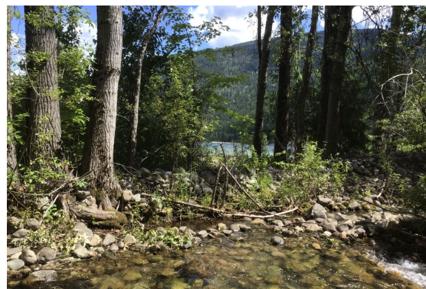
F) DHL-FP-08: Looking east at the left bank dike, approximately 150 m downstream of Lower 6 Mile Road.
