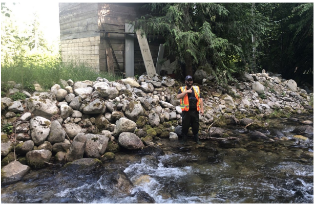
C) DHL-FP-04: Placed creek bed material on left bank approximately 180 m upstream of Highway 3A.
