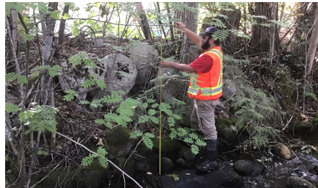
D) DHL-FP-11: Approximately 80 m upstream of Highway 3A looking at left bank with 1 m boulders. Similar sized material was observed on right bank (DHL-FP-10).
