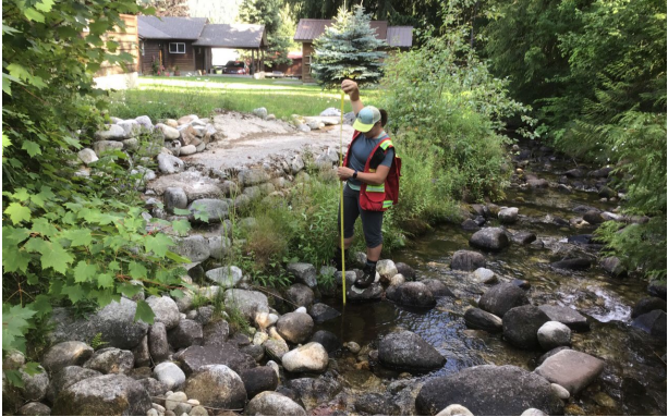
A) DHL-FP-10: Concrete wall on left bank, approximately 30 m downstream of bifurcation structure looking downstream.
