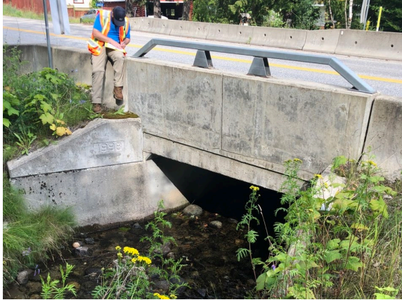
A) Looking downstream at Duhamel Highway 3A East Bridge.
