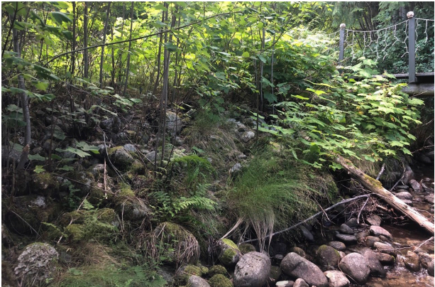
B) DHL-FP-15: Looking at left bank, just upstream of Pedestrian Bridge 2 (right side of photo).
