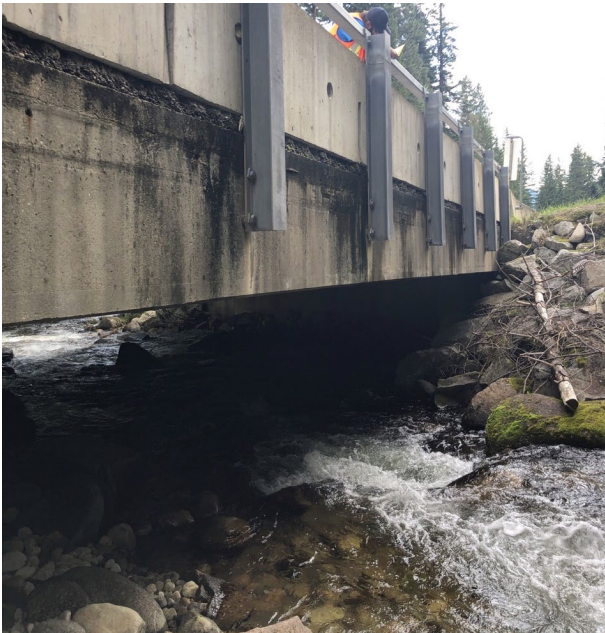
C) On upstream left bank looking at right bank riprap armoring under Duhamel Highway 3A West Bridge crossing the western channel.
