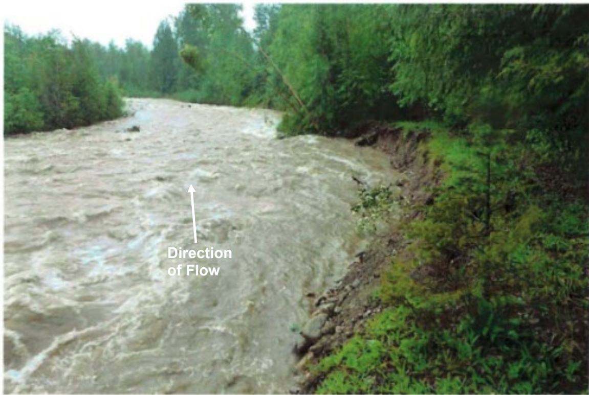
Figure 3-7. June 25, 2013 photo of erosion of a historical berm, 1 km north of Highway 3A (BC MFLNRO, 2013).
