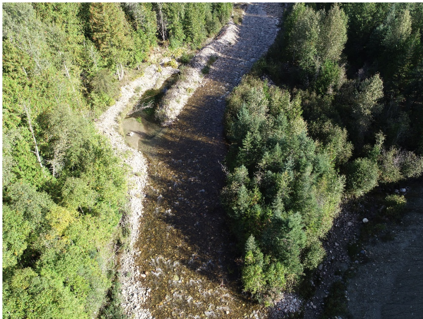
Photo 20. Dyke along Crawford Creek's west bank, 600m north of Highway 3A. Photo: Explore, September 25, 2019.
