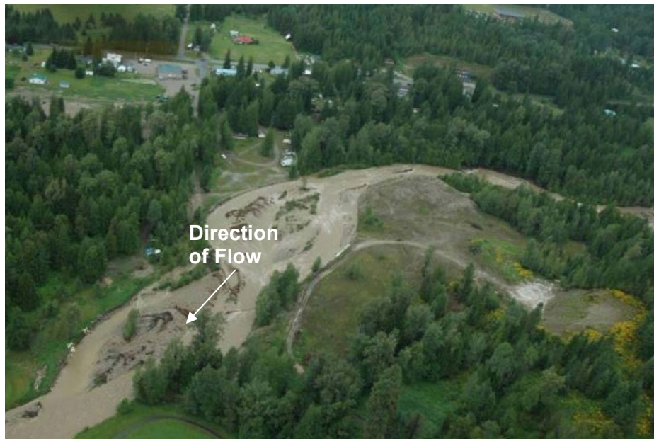
Figure 3-1. 2013 Flooding of Crawford Creek 500 m north of Highway 3a. Photo: BC Ministry of Forest, Lands and Natural Resource Operations (2013).
