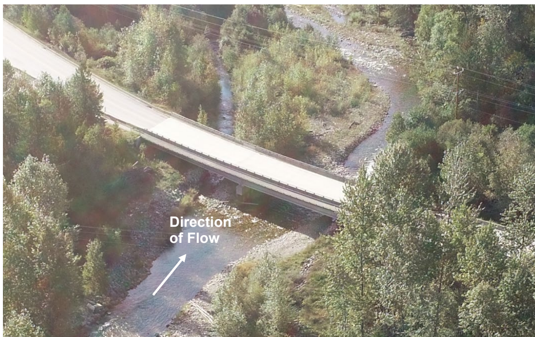
Figure 3-4. Drone photo of Highway 3A bridge. Photo: Explore Survey Inc, September 25, 2019.
