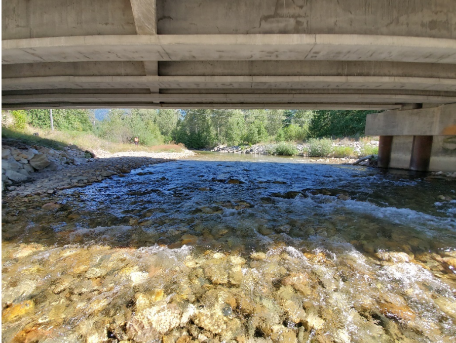
Photo 17. Looking upstream under Highway 3A Bridge, Photo: Explore, August 18, 2019.
