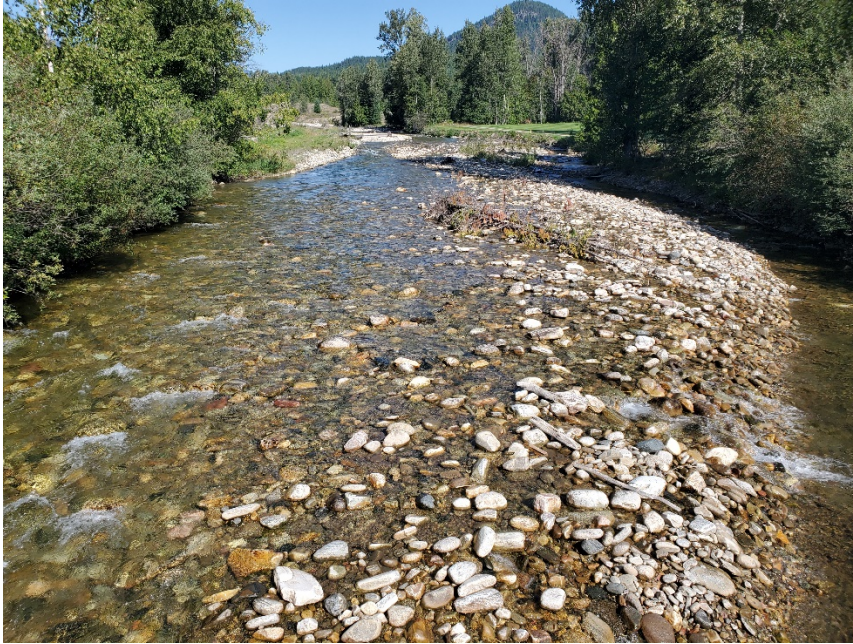
Photo 15. Looking upstream of Pedestrian Bridge crossing Crawford Creek, 200 m north of Highway 3A. Photo: Explore, August 18, 2019.
