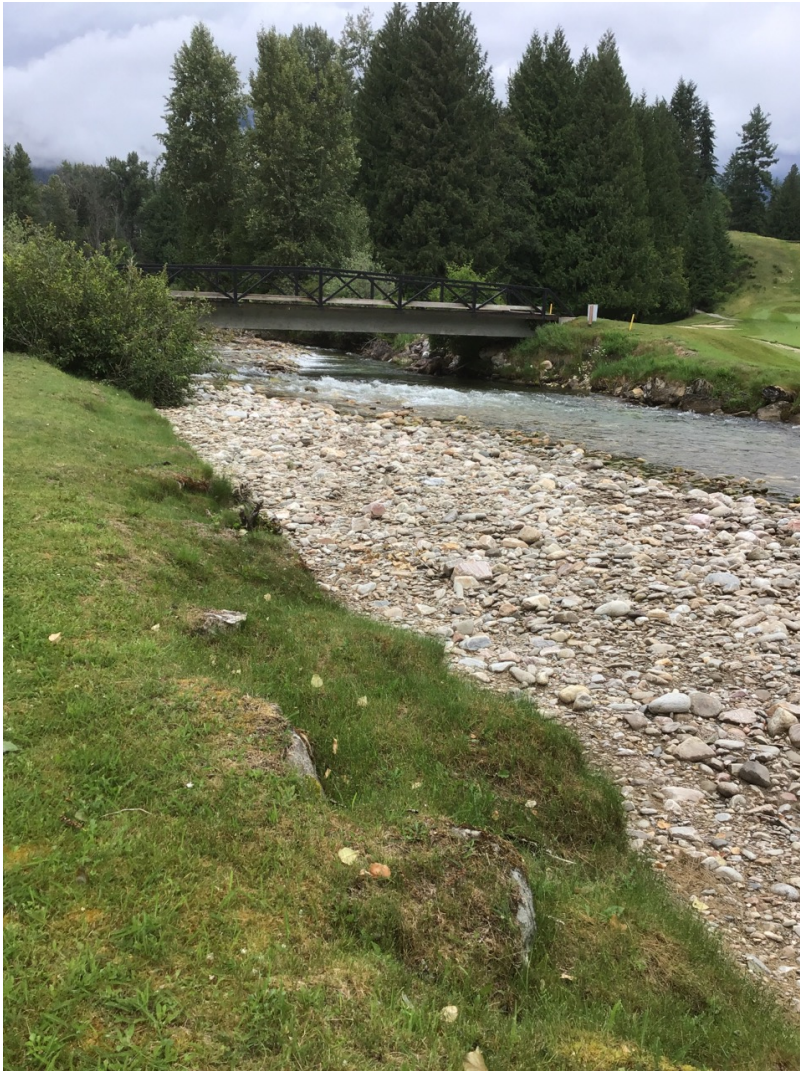
Photo 10. Pedestrian Bridge crossing Crawford Creek, 200 m north of Highway 3A. Photo: BGC, July 4, 2019.
