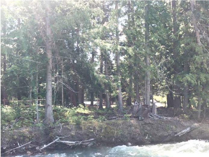
Photo 20. Standing on the left bank bar looking across to right bank (flow is right to left) at bank erosion approaching fence line, approximately 300 m upstream of the mouth. Photo: BGC, July 25, 2019.
