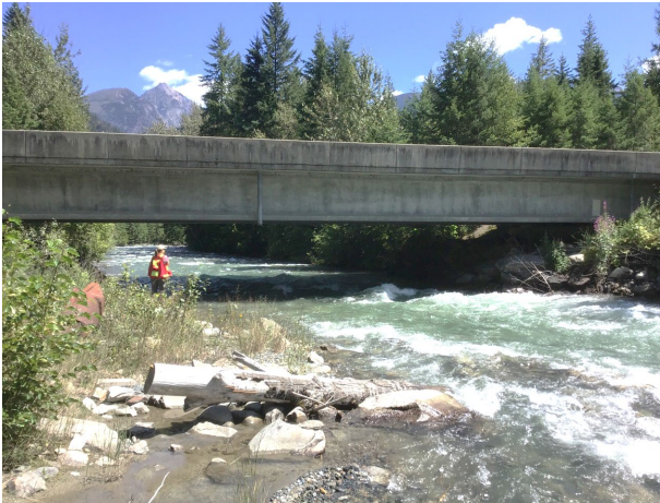
C) Looking at Cooper Highway Bridge from upstream left bank.
