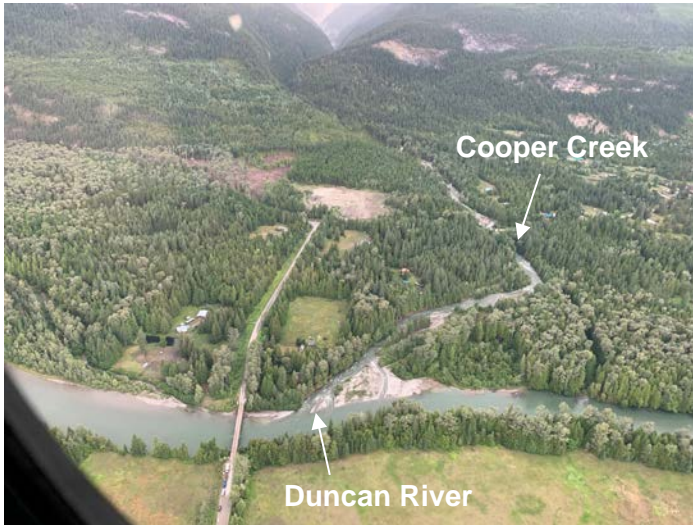
Photo 1. Overview photo taken during helicopter overflight looking west at Cooper Creek discharging into Duncan River. Photo: BGC, July 6, 2019.
