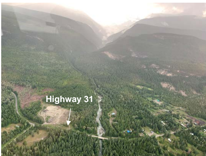
Photo 3. Overview photo taken during helicopter overflight looking west at the Cooper Creek fan-delta with Highway 31 crossing Cooper Creek. Photo: BGC, July 6, 2019.
