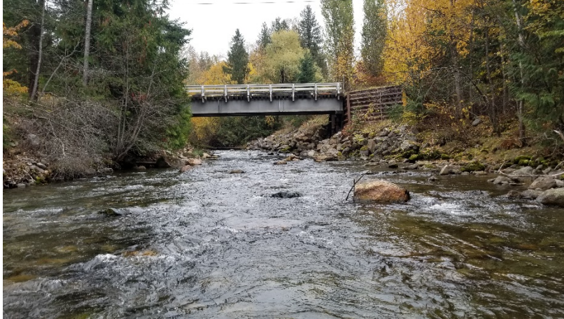
Photo 7. Downstream McCormack Bridge looking upstream. Photo: Explore Inc., October 23, 2019.
