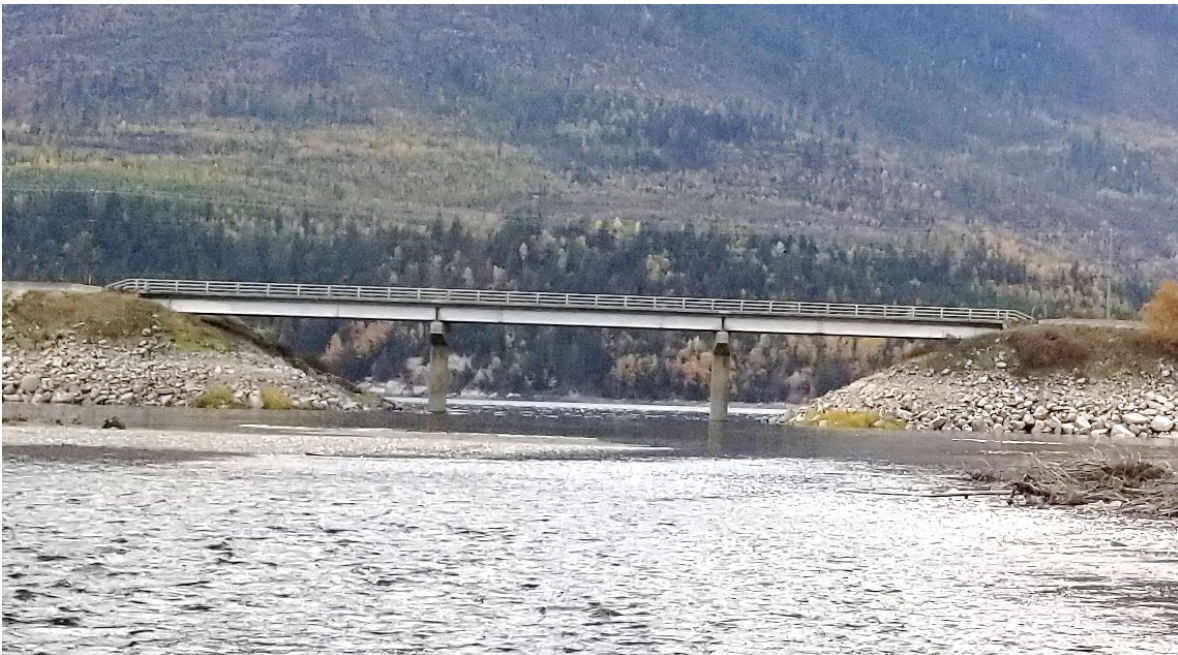
Figure E-12. Upstream of the Highway 6 bridge looking west towards Lower Arrow Lake. Photo: Explore, October 19, 2019.
