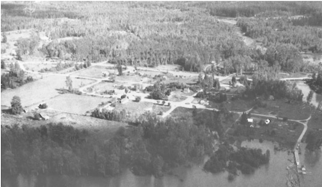
Figure 3-1. The Burton Wharf from the air, during high water. Photo: Arrow Lakes Historical Society.
