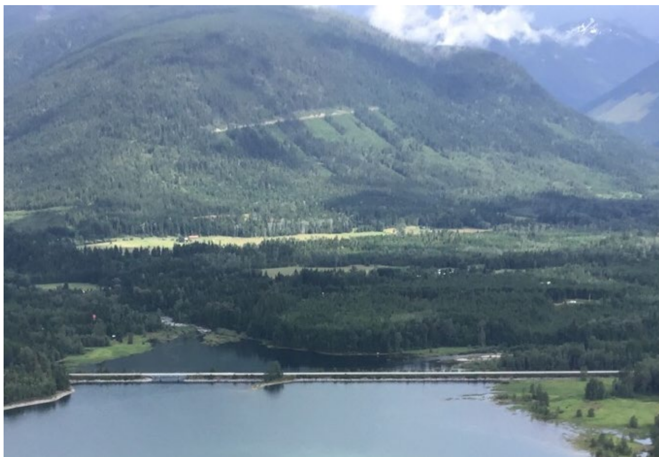
Figure 3-4. View looking east of the embankment and bridge along Highway 6 with Lower Arrow Lake in the foreground. The outlet of Caribou Creek is on the left and the outlet of Burton Creek is on the right. BGC, July 6, 2019.
