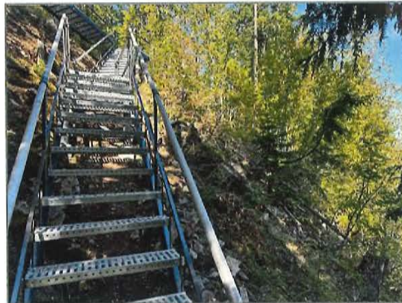
Photo 8. View of constructed metal grate stairway and deck (July 26, 2023).
