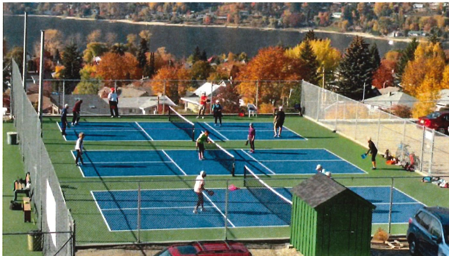
Nelson Tennis Club – Phase 1 completed works – 3 Pickleball Courts
