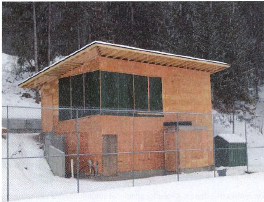
Phase 2 – Facility Centre Complex – to lock up
